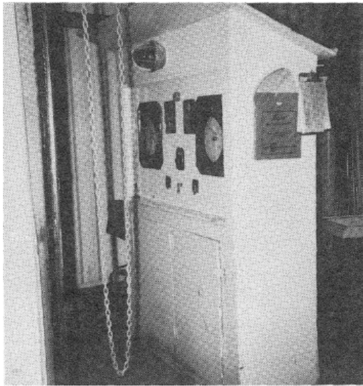
Figure 1. Ethylene Oxide Control System Circa 1950's.
